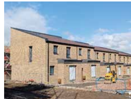
12 Progress at Hamiltonhill
